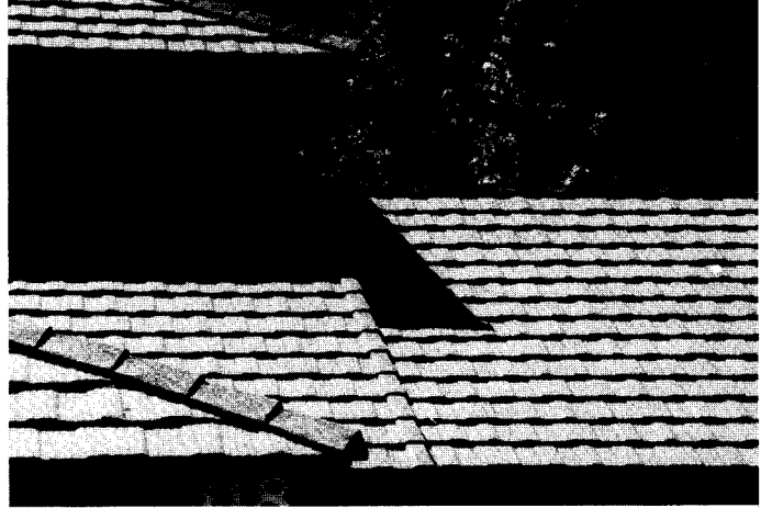
Photo 4 Metal simulating wood shakes.
