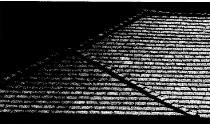
Photo 9 Fiber cement simulating slate.
