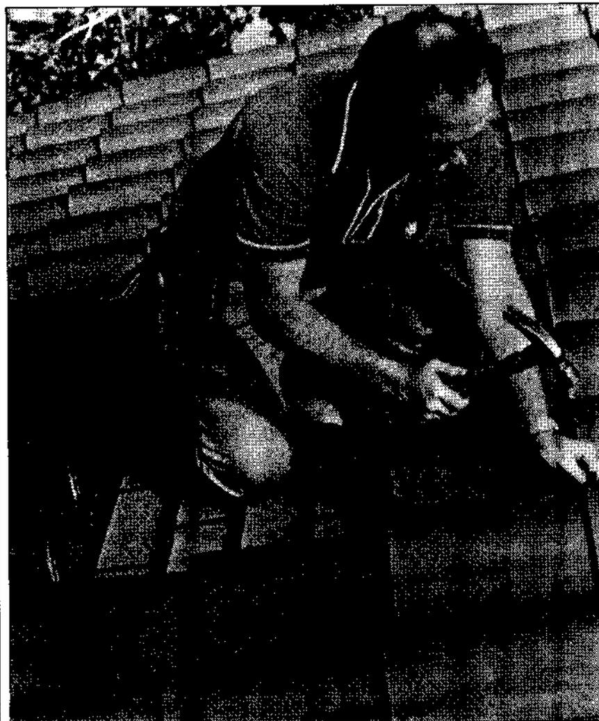
Metal steep roofing is available in a variety of shapes. This aluminum zinc coated style from Metal Sales Manufacturing Corp. simulates clay tile.
