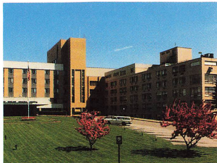
An important Sarnafil roof protects New England Memorial Hospital, Stoneham, Massachusetts.
