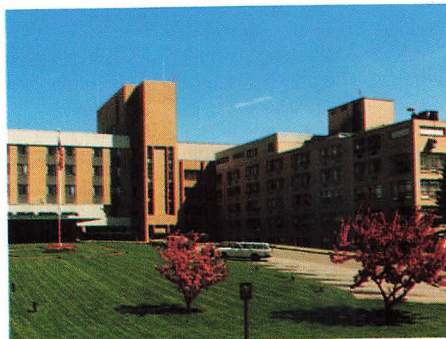
An important Sarnafil roof protects New England Memorial Hospital, Stoneham, Massachusetts.
