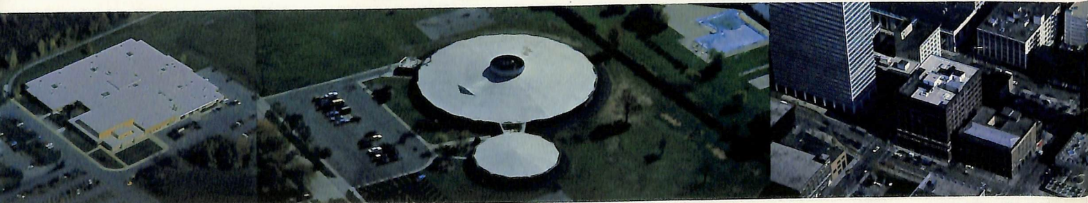
Dickinson Center and Cass School, Livonia, Michigan. Single Ply International (Livonia, MI). Marquette Building, Detroit, Michigan. WBC Roofing (Detroit, MI).
