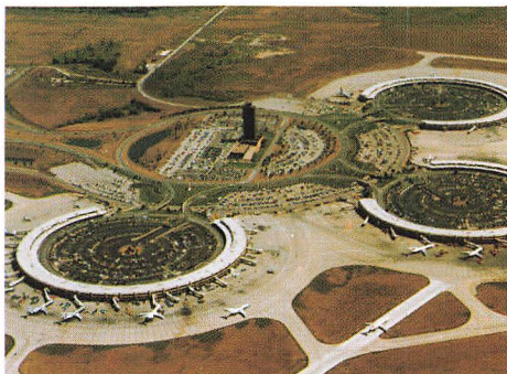
An important Sarnafil roof protects the Kansas City International Airport Terminal.
