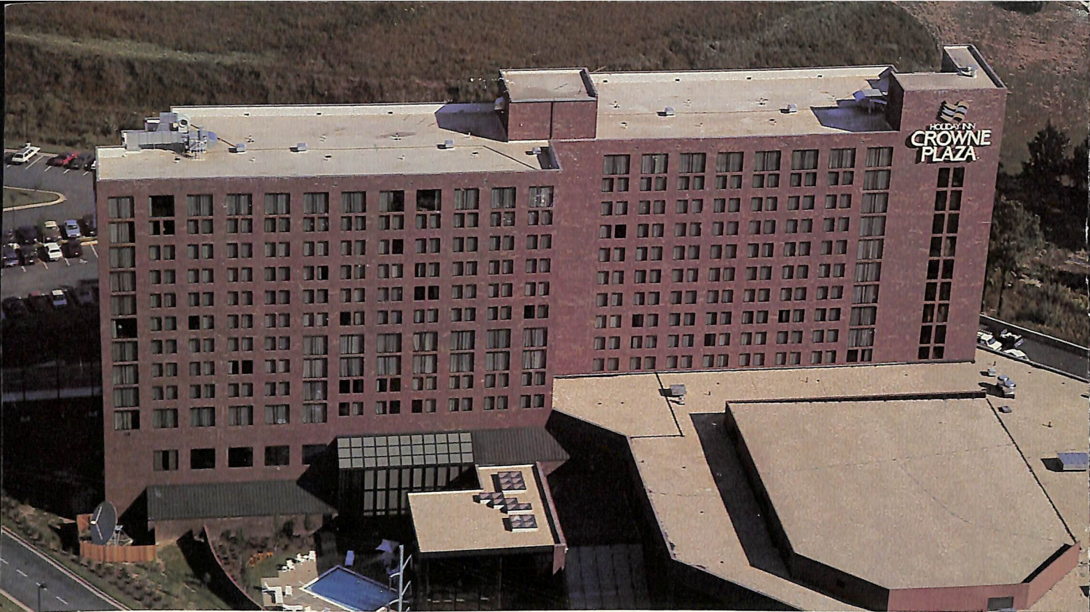
Holiday Inn/CROWNE PLAZA, Atlanta, Georgia. Southeastern States Roofing (Orlando, FL).
