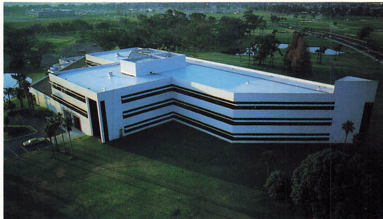
Hi-Tuff tops the home of Critikon, Inc., a Johnson & Johnson company.
