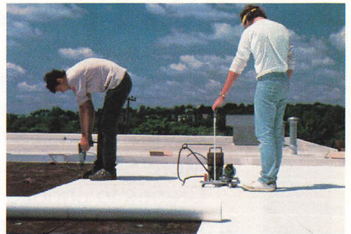
CoolTop's mechanical attachment and heat welding system mean faster installation.
