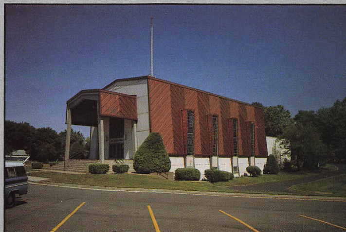
Project: First Christian Church, Henderson, KY Contractor: Artisan Sheet Metal Corp., Evansville, IN
