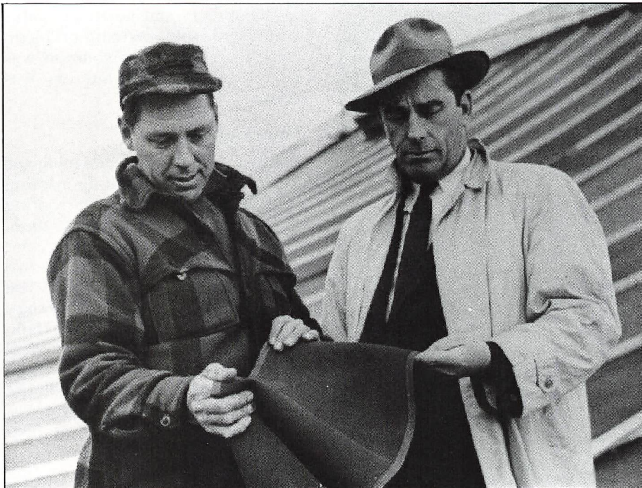
Workmen inspect a piece of the neoprene they used to roof Yale's Ingalls Ice Arena.
