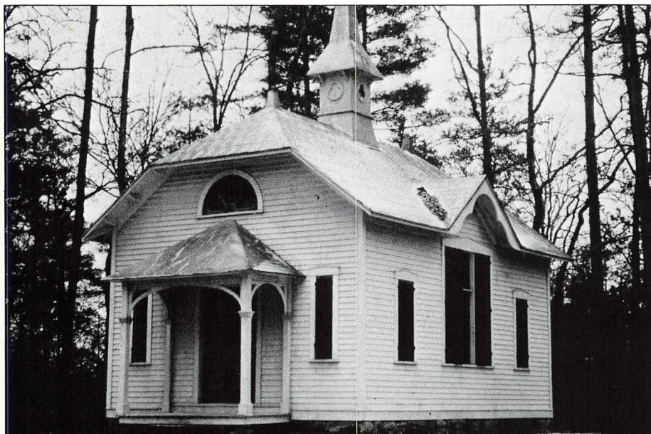
The Hughes Public Library, built in 1882, had a standing seam and stamped sheet metal roof before restoration.
