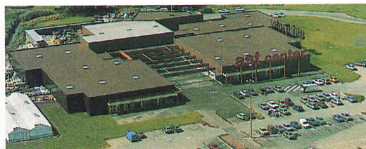
Waterproofing of industrial building
