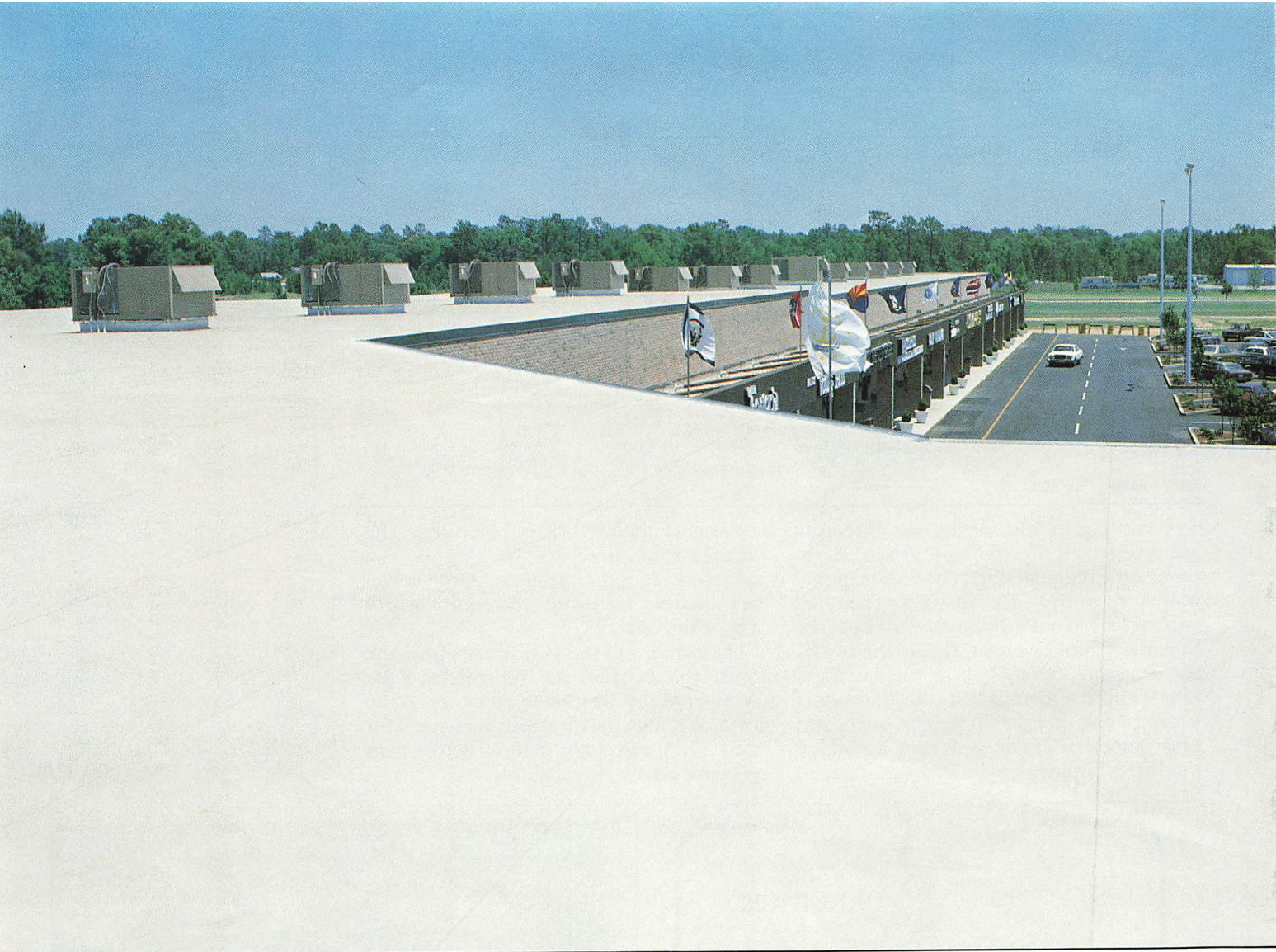
Mill Store Plaza/Valdosta, Georgia. Contractor: Bi-State Roofing/Lakeland, Georgia
