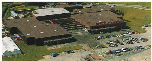
Waterproofing of industrial building
