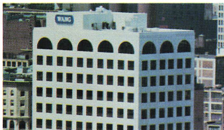
Sarnafil roof on Wang Laboratories' Boston facility.
