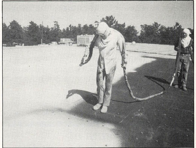
Spraying Polyurethane Foam.
