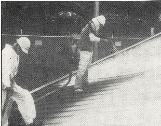
Spraying Polyurethane Foam on Metal Roof Deck. (U.S. Navy photos)
