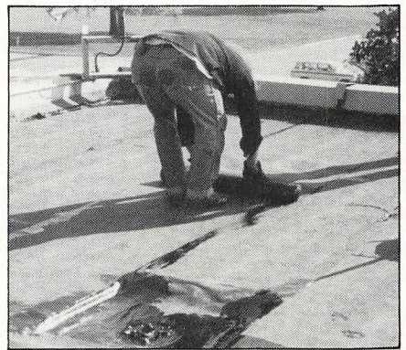
Figure 3: Hot-mopped polyester roof
