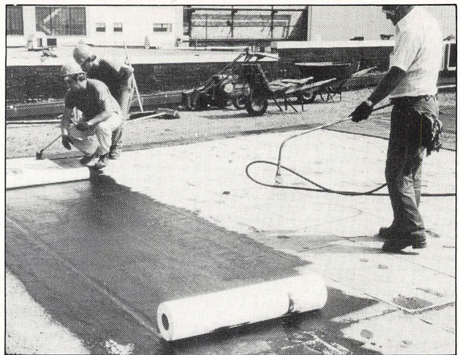
Figure 1: Applying a polyester system
