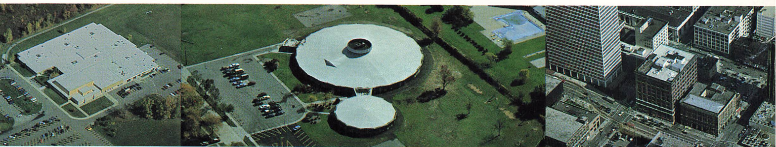
Dickinson Center and Cass School, Livonia, Michigan. Single Ply International (Livonia, MI). Marquette Building, Detroit, Michigan. WBC Roofing (Detroit, MI).
