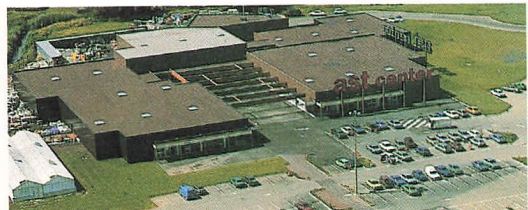
Waterproofing of industrial building
