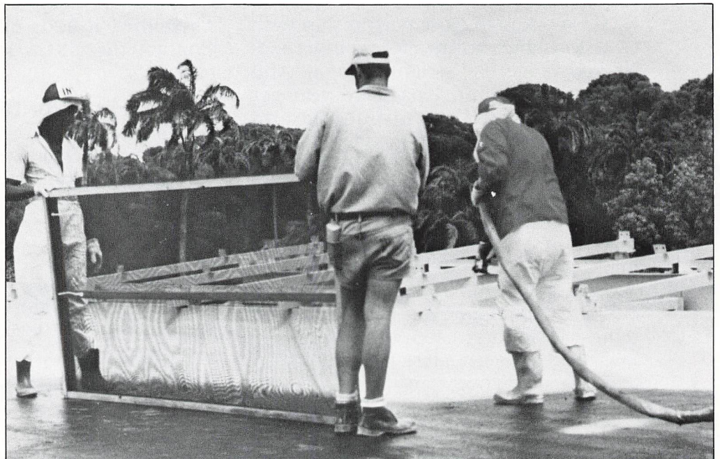
Workers from Sunpower, Ltd. in Bridgetown apply urethane foam insulation system to new insurance company building.
