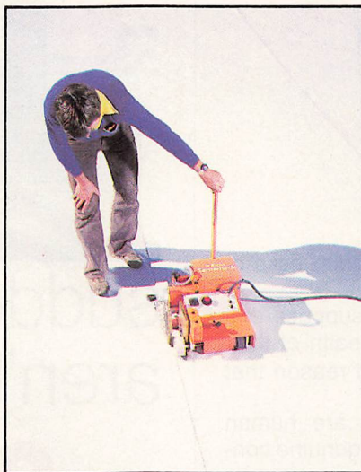
Sarnafil roofing requires no adhesive or sealants at the joints. Material is fused by means of hot-air welding to produce a continuous leak proof membrane.
