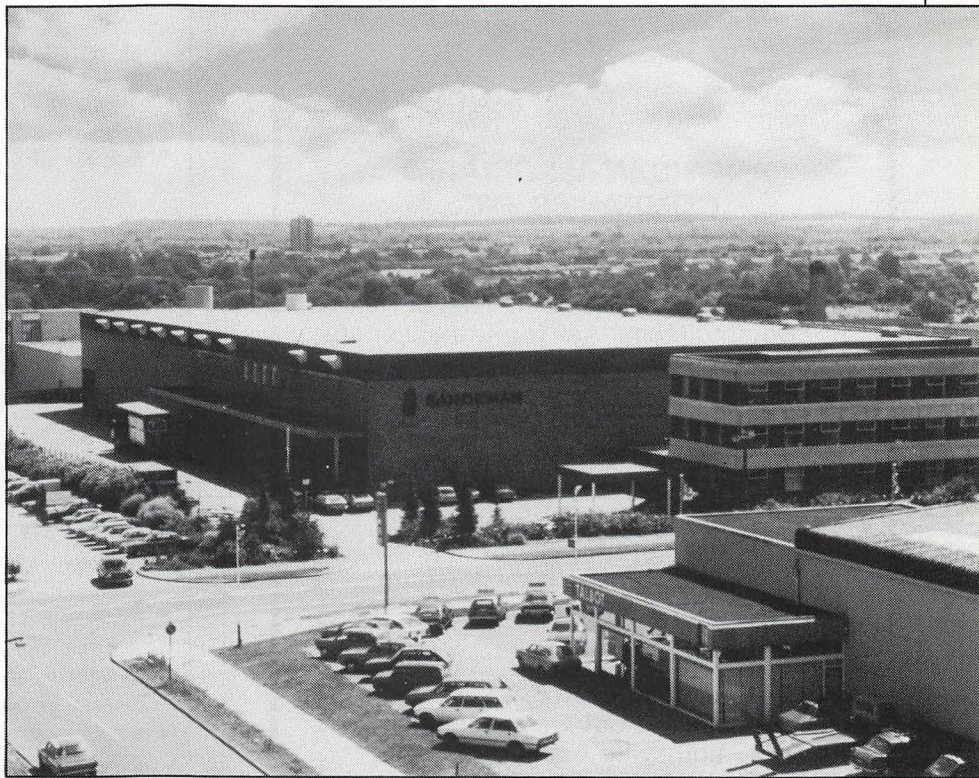
Top , An example of an original roofing felt manufacturing machine circa 1894 by Jens Villadsens Fabriker, Denmark. Bottom , The 6,000 square meters of roof at Sandeman Wine Merchant's distribution center in Harlow, Essex, which has been refurbished with Derbigum high performance roofing.
