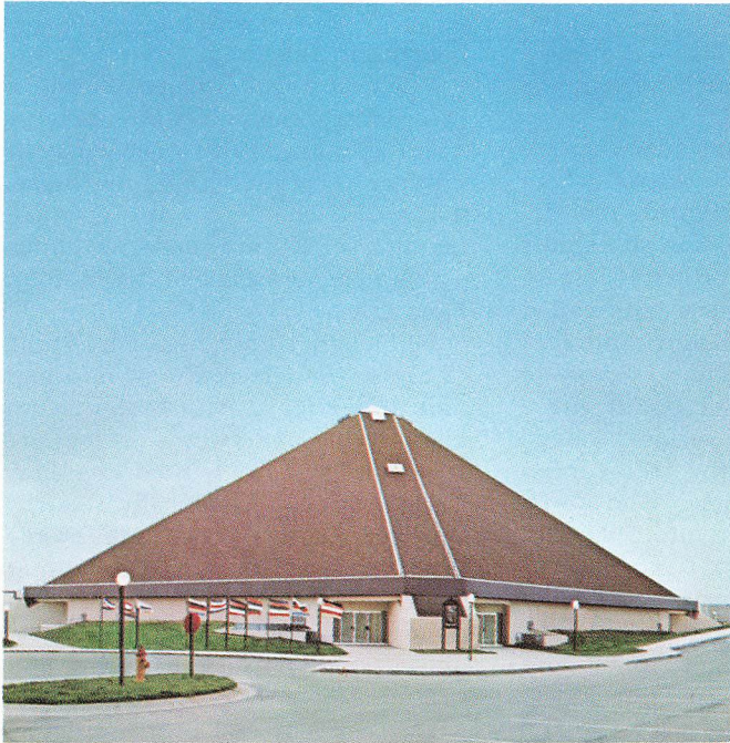
Project: John Knox Village International Pavillion, Lee's Summit, Mo. Architect: Environmental Design Association
