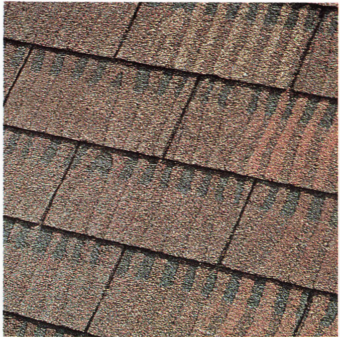
Roofing Contractor: West-Bar Co./Allen Meyers Co. (Joint Venture), Kansas City, Mo.
