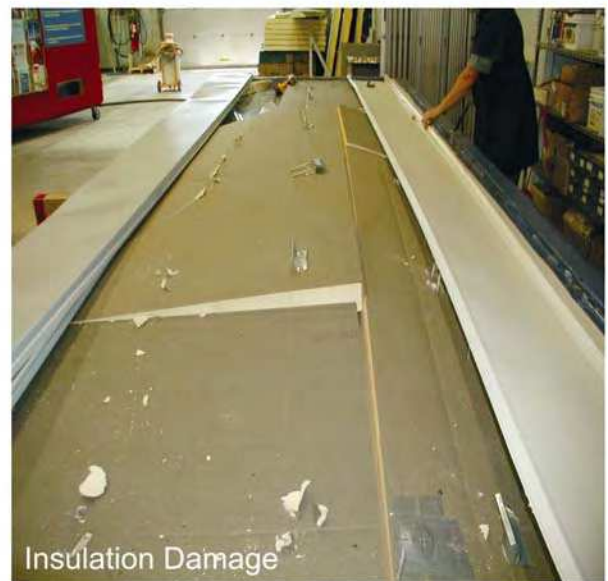
Panel Seam Separation
