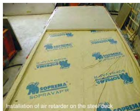
Figure 9: Typical layout of assembly with air retarder
