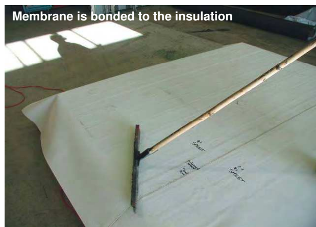
Figure 5. Mock up Construction Process of FBA with Barrier
