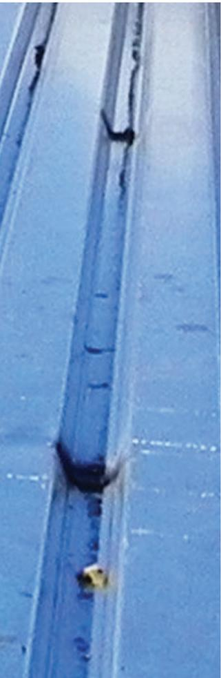
nonuniform uplift loading conditions, such as those created with seam-fastened mechanically attached single-ply membrane roof systems. SDI's design guidelines are based on uniform loading, such as those provided by an adhered membrane roof system.
