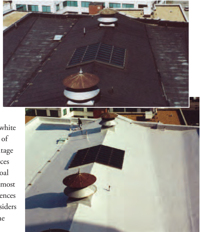
A 14-year-old built-up roof system before and after coating. The roof, coated in 1996, was recoated within the next five years to extend the coating's life.
