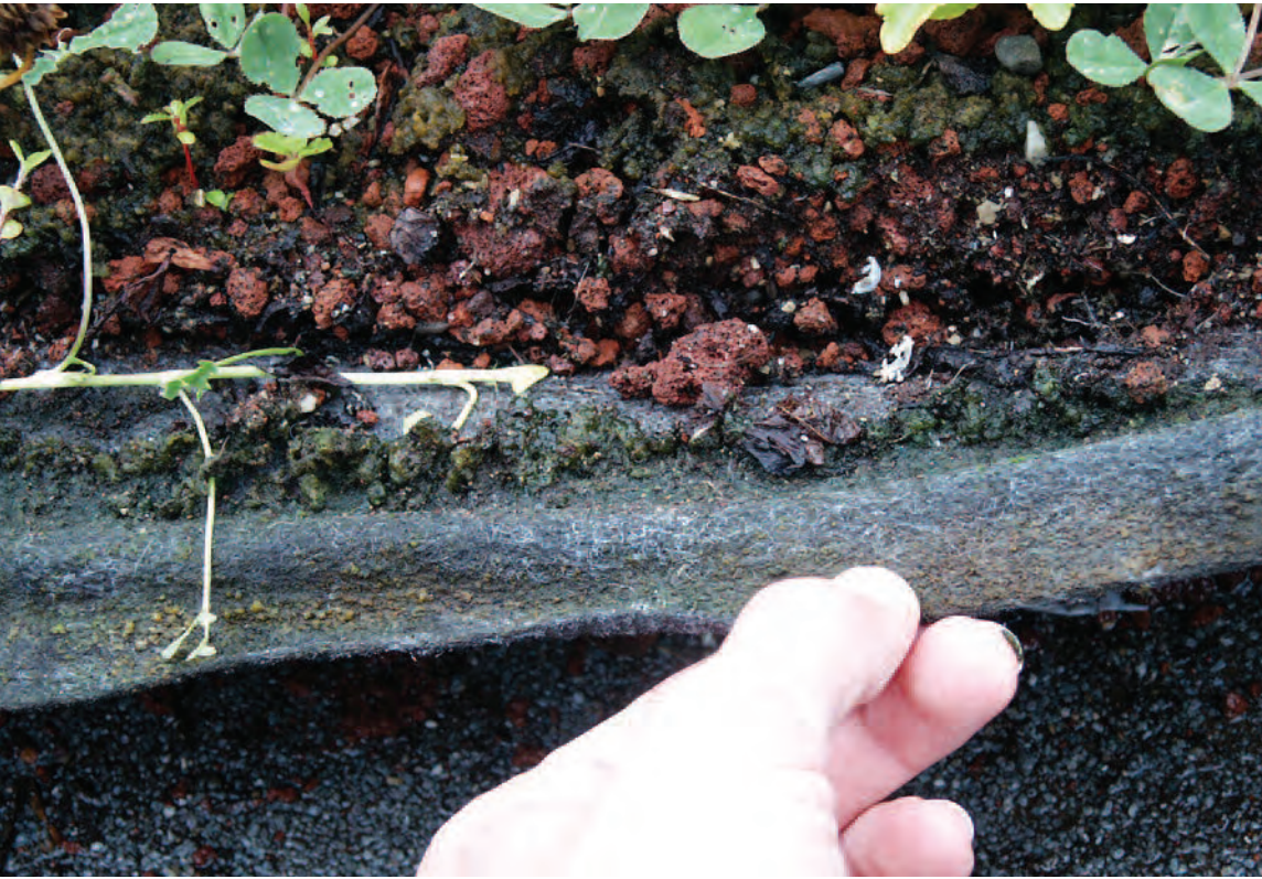
Photo 2: This filter fabric is covered with a thin layer of growth medium and plantings.
