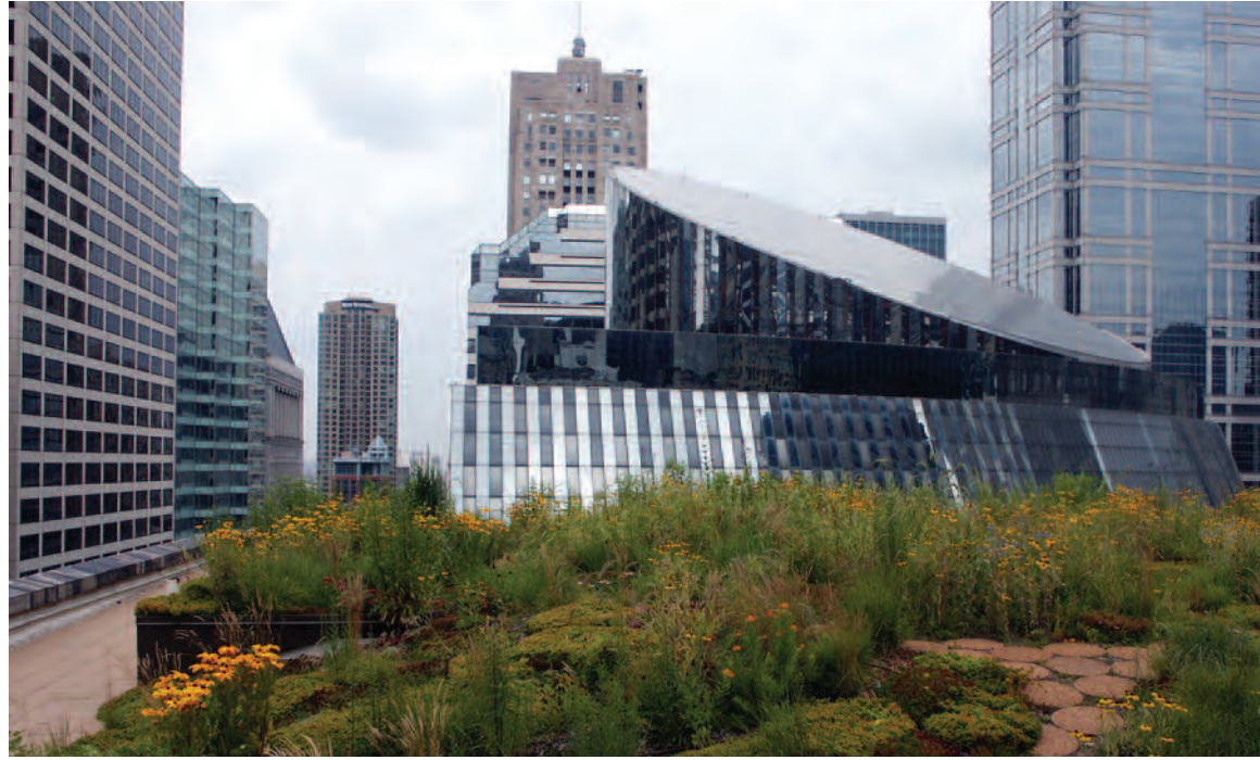
Photo 3: The vegetative roof system atop Chicago's City Hall
