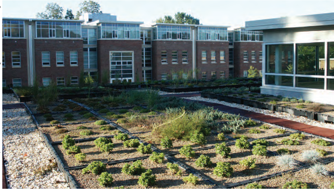
Photo 1: The Jordan N. Carlos Middle School Art Building at Woodward Academy, Atlanta, features a vegetative roof system within trays elevated above the roof membrane.
