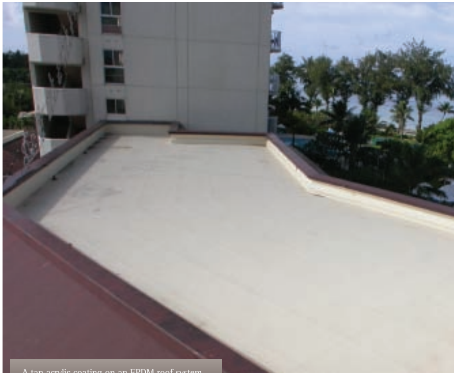
A tan acrylic coating on an EPDM roof system
