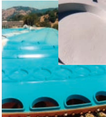
Polyurethane can provide waterproofing and lasting color in a fluid-applied roof coating system.
