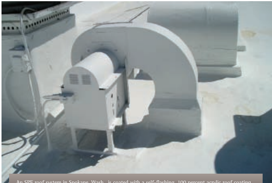
An SPF roof system in Spokane, Wash., is coated with a self-flashing, 100 percent acrylic roof coating.
