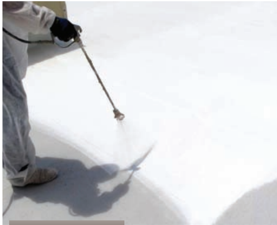
Coating is spray-applied on a roof system.
