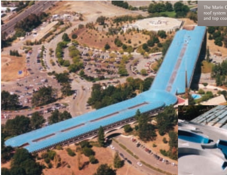
An aliphatic polyurethane top coat was applied over a urethane base coat.
