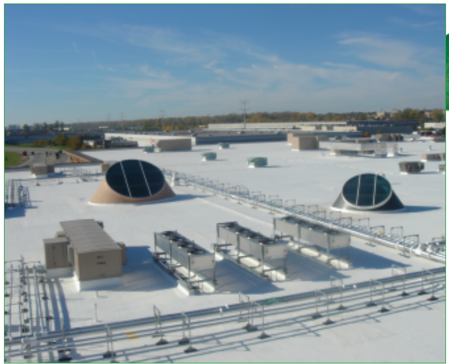
This smooth 2,600-square-foot built-up roof system on KV Pharmaceutical's building in St. Louis was restored with a biobased coating.
