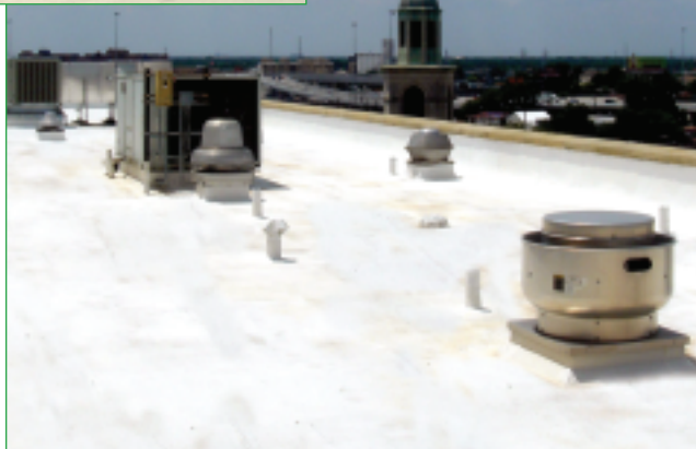
Before (top left) and after (bottom right) photos of the roof system restoration with a biobased coating on Baptist Medical Center's surgical wing in San Antonio. Photos courtesy of Green Products LLC, Romeoville, Ill.
