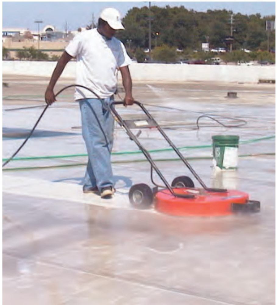
For proper adhesion, a roof substrate must be cleaned and prepared satisfactorily; most roof surfaces are best cleaned by power washing.
