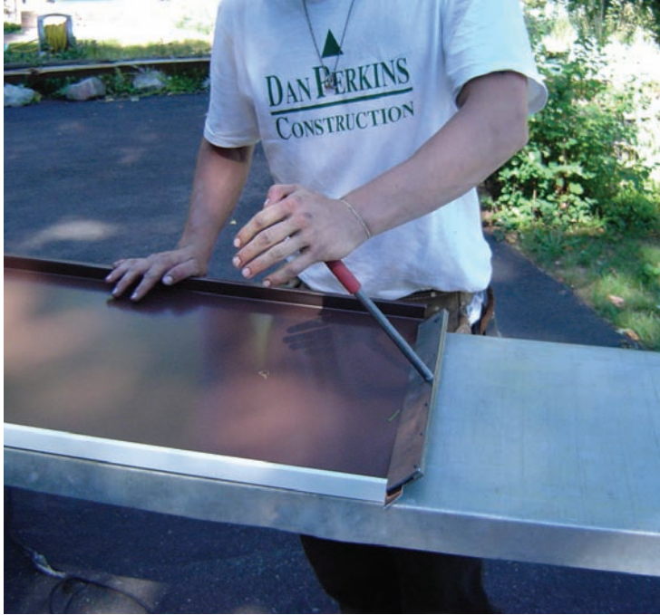
The roofing pans are “box panned” before they are installed into the ridge, and baffles are applied to prevent wind from driving water and snow directly into the perforations in the C channels.
