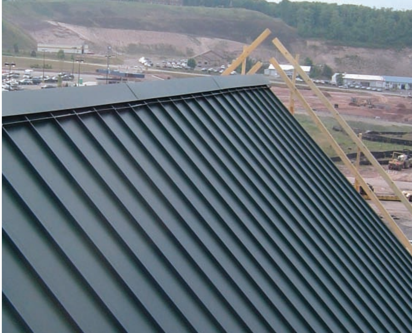
The ridge vent and cap shown are designed to be installed before the roofing panels are installed. This has proved to be a watertight system that can be applied more efficiently and safely than ridge caps that are installed after panel installation. Photos courtesy of Dan Perkins Construction Inc., Ishpeming, Mich.
