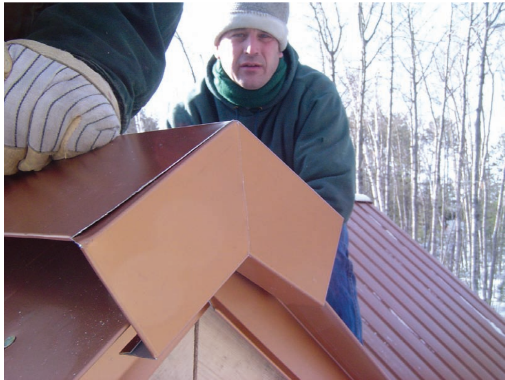
The ends of the ridge are closed with an end cap that is slid into the hem holding the cap to the perforated C channels.
