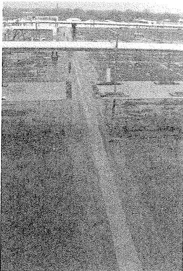
A zero profile expansion joint installed in a Built-Up-Roof
