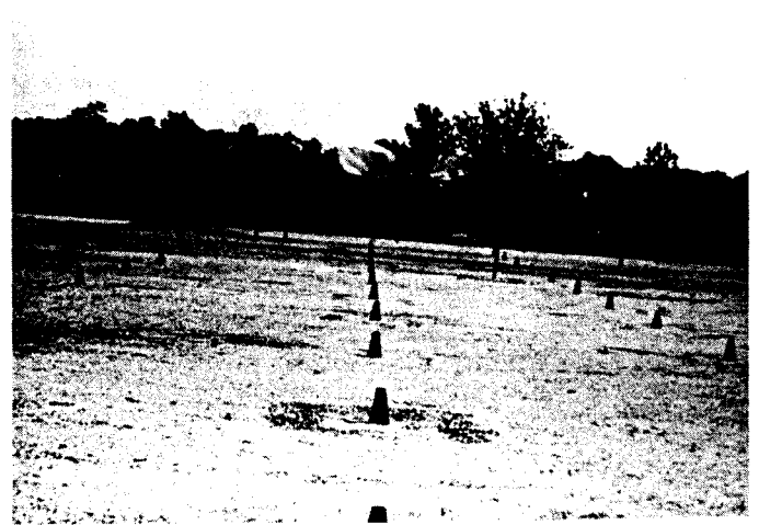
FIGURE 4 A roof containing numerous breather vents as recommended by current industry standards. (Photo from the RIEI collection.)
