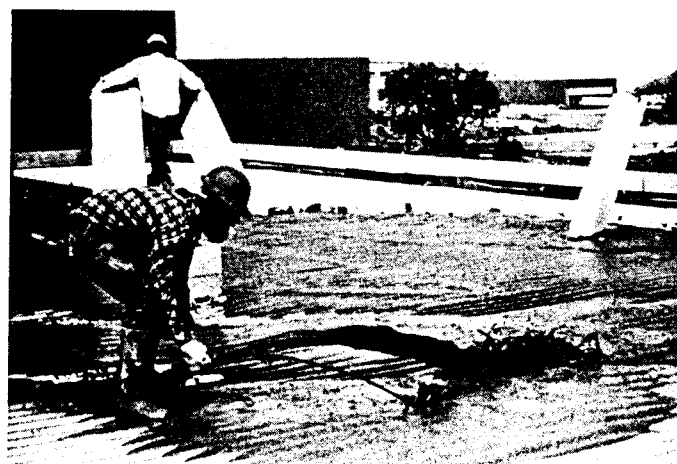
FIGURE 2 Placing a wet-applied insulation (Photo from the Roofing Industry Educational Institute Collection).
