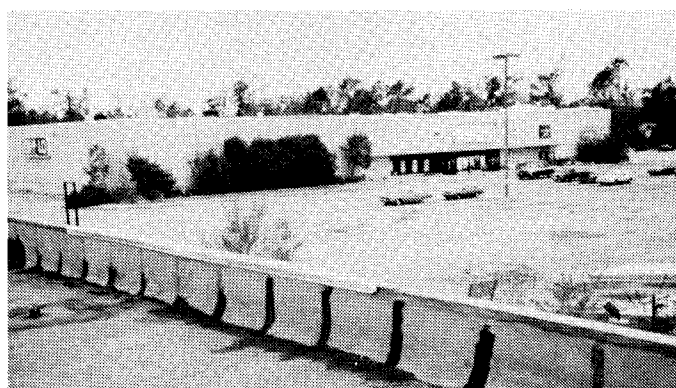
Photo 6 Ten foot long (3 meter) sections of 0.023-inch (60 millimeter) aluminum coping were attached with only two nails at each end. The coping had 2½-inch (62 millimeter) vertical legs. Most of the coping sections blew off.
