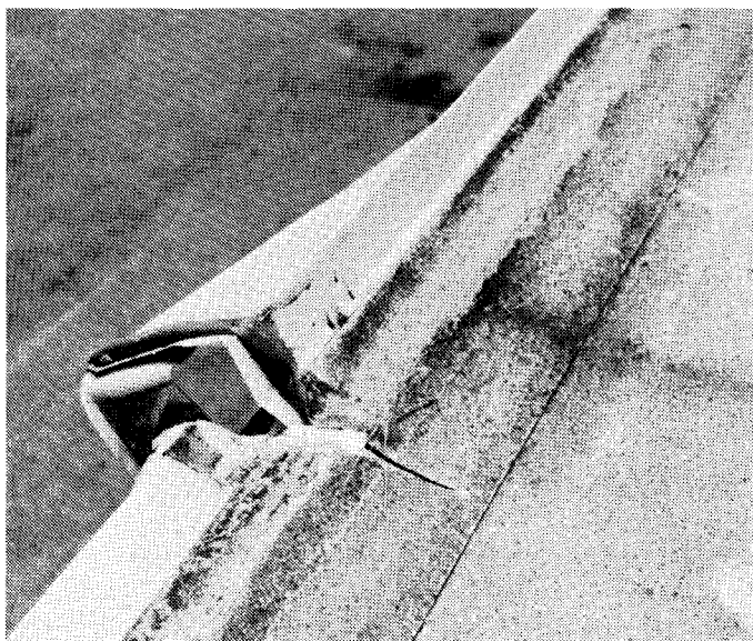
Photo 3 Good cleat attachment and cleat/metal edge flashing interlock prevented the metal edge flashing and membrane from lifting and peeling.
