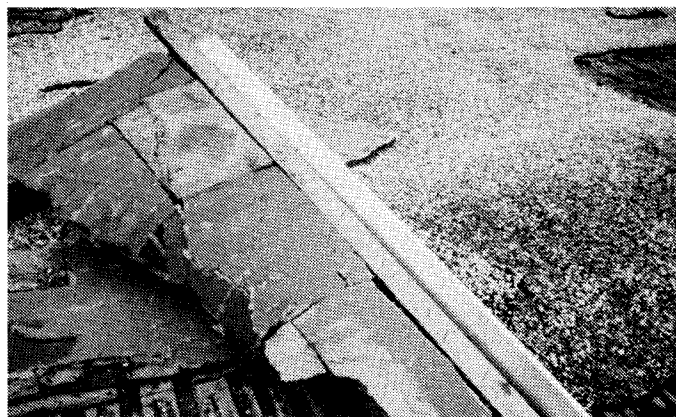
Photo 5 Metal edge flashing attached to a nailer, which was nailed to a bottom nailer that was bolted to the wall. The nails attaching the top nailer had a calculated working load capacity of 90 pounds per lineal foot (124 kilograms per meter).
